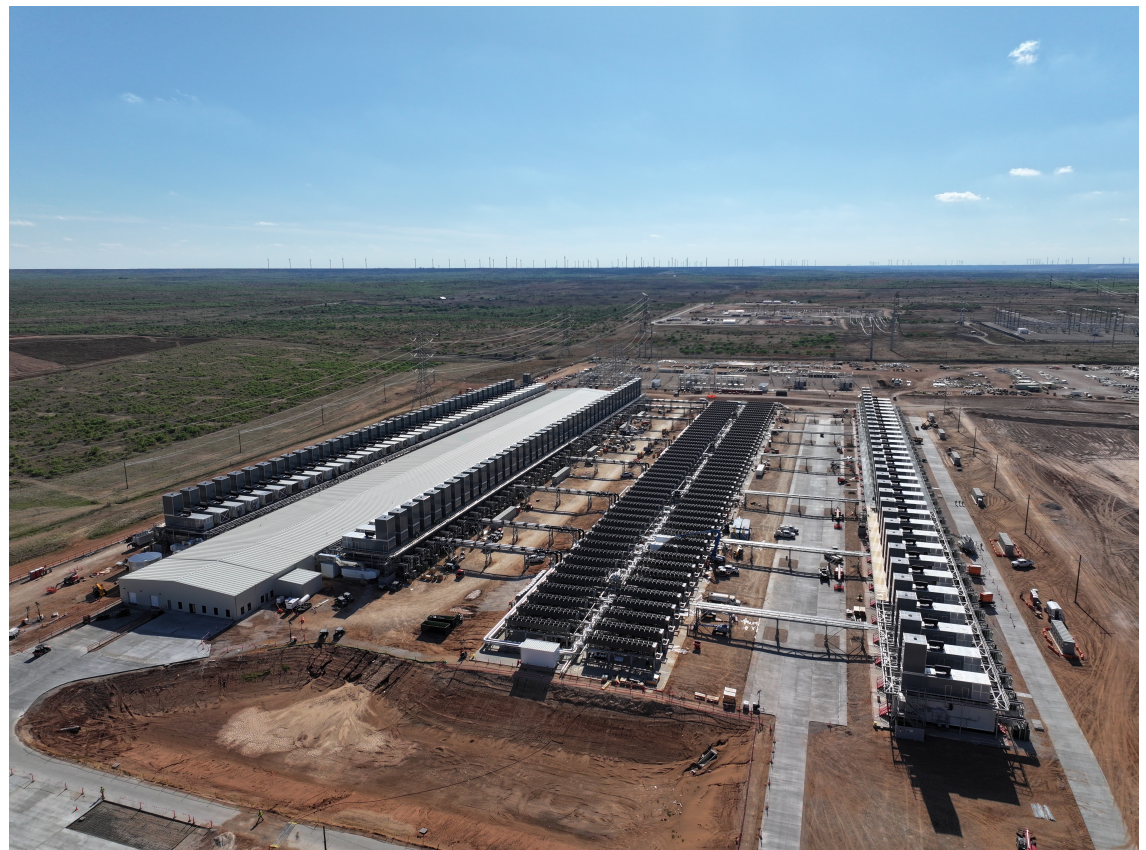
Galaxy's Helios Data Center campus under construction for Phase I, April 2026.
